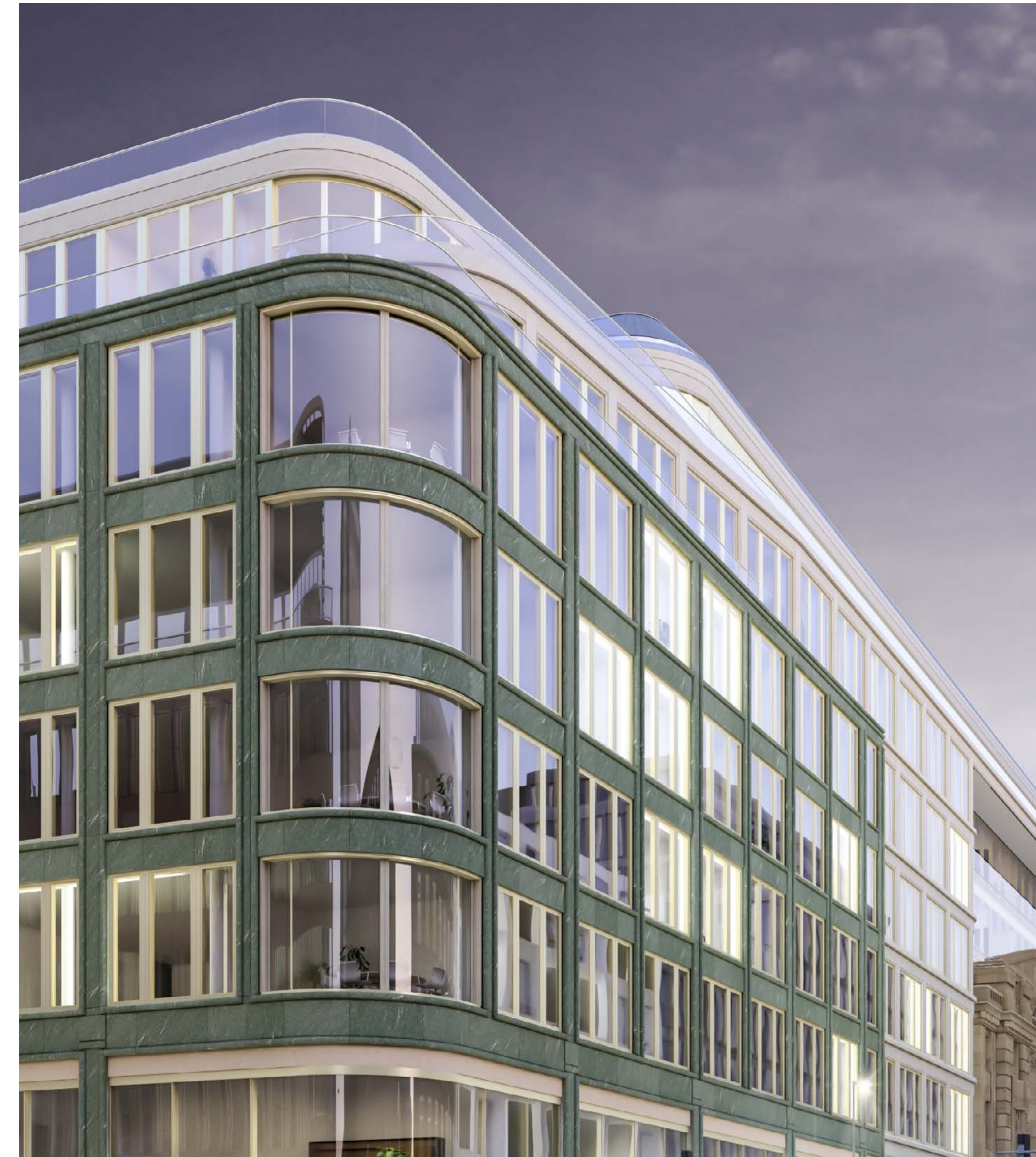
The move to the new Dusseldorf office premises, which has been awarded platinum pre-certification by the German Sustainable Building Council, is scheduled to take place in 2027.
